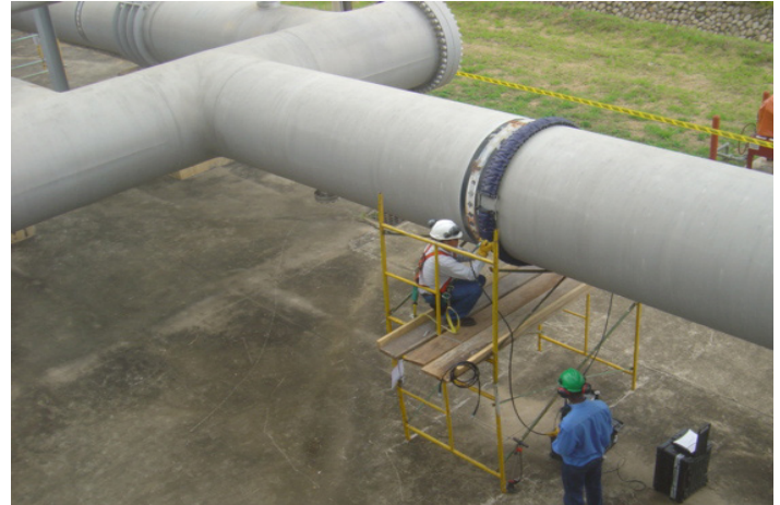
A "Slug Catcher" being inspected by a 48" combined inflatable ring.
