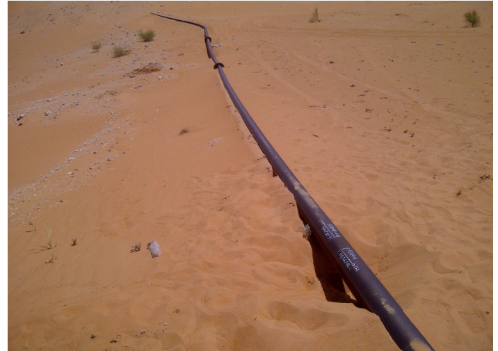
An overview of 6" flow line.
